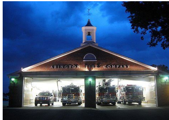
Figure 2 Station 100 Abington Fire Company
